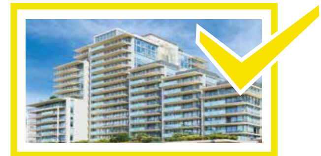
Hotels, hospitals, residential complexes
