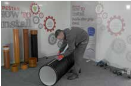
2. Determining position for montage
