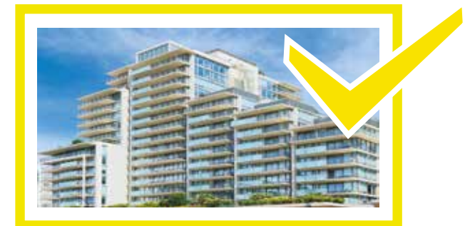
Hotels, hospitals, residential complexes
