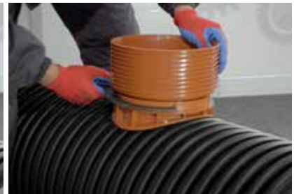
12. Final tightening of sag
