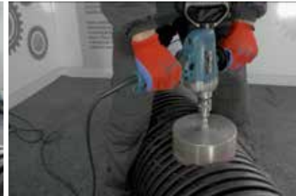
4. Drilling holes with crown saw
