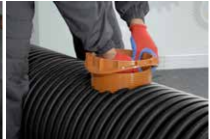
8. setting the spacer ring
